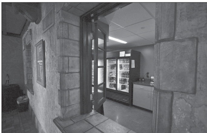
The concessions area improvements include new coolers.
